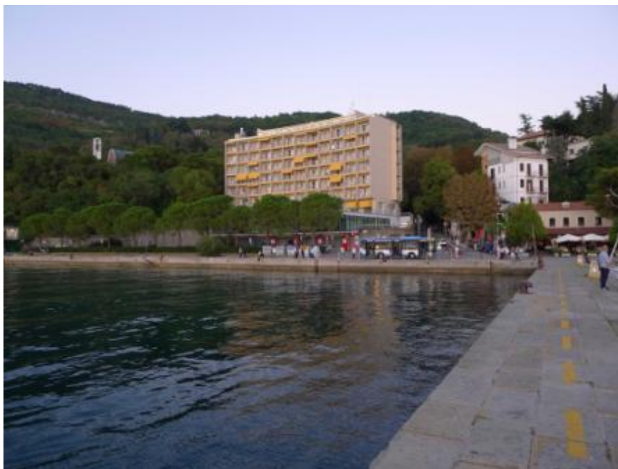
ICTP accommodation and teaching block, Trieste, Italy
